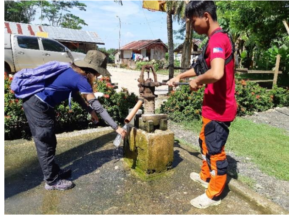
Individual jetmatic pump used to get potable drinking water located in Purok 6, Brgy. Dakutan. GPS Coordinates: 8° 38' 53.44" N, 125° 40' 39.50" E
