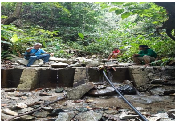
Photo shows a concrete box installed to the surface water source (creek) of Barangay San Isidro. It supplies 5 Puroks (1, 2, 3, 4, and 5) of the Barangay and is mainly used for drinking. The water never dries out but is turbid during heavy rains and rainy season. GPS coordinates: 8° 28' 45.0717" N, 125° 58' 30.2978" E.
