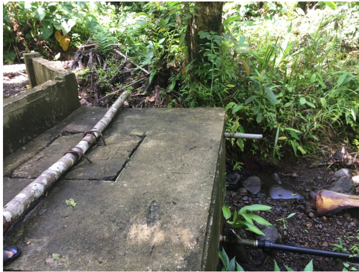
Photo 1. Source 1 of Barangay Bagacay is connected to Anaub Creek, water distribution is 50% level 3 and the remaining is still at level 2 system. This source served as drinking water of the entire barangay, and constructed by year 2015 and funded by the KALAHI. It gets turbid when heavily rains and insufficient during dry season.
