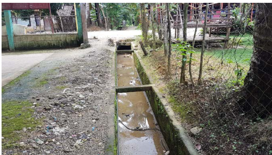
Figure 2. Heavily silted drainage canal near the barangay gym located in Purok 6 in Barangay Lago. The congested canal is the main contributor of flooding within the barangay.
