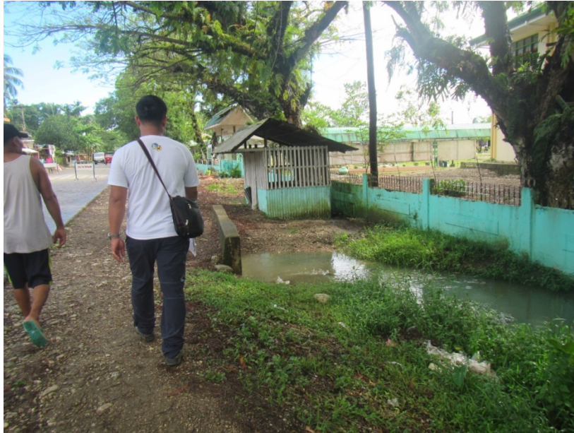
Figure 11. Drainage canal in Brgy. Hornasan near Sto. Niño National High School is not sufficient and may cause localized flooding in the area.
