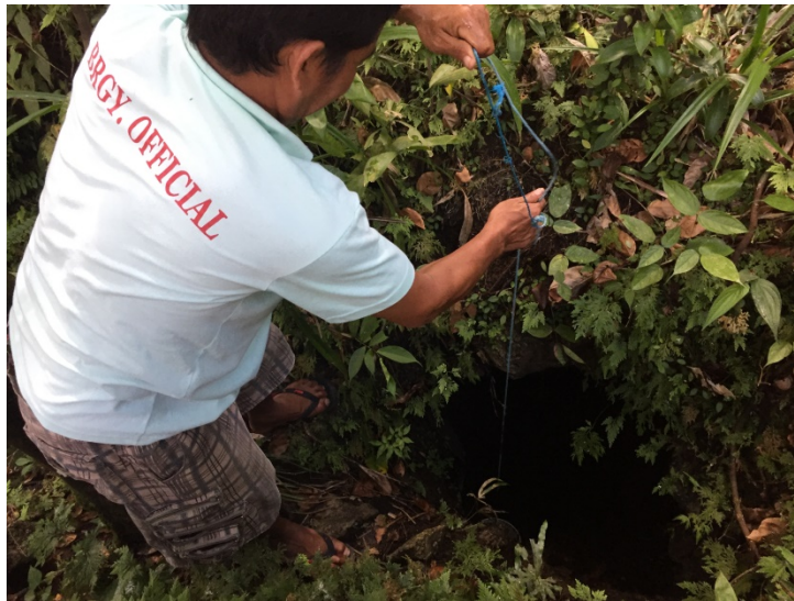
Photo 2. This spring source within a sinkhole is the proposed water source of Barangay Mabuhay and it is still on-going construction. It has an estimated depth of 2.5 to 3.0 meters from ground to water level.
