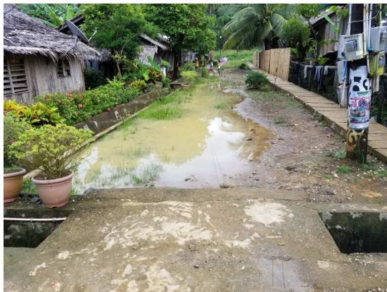
Figure 6. Confined meteoric water in the passageway of Purok 2, Brgy. San Antonio and the established drainage canals surrounding it.
