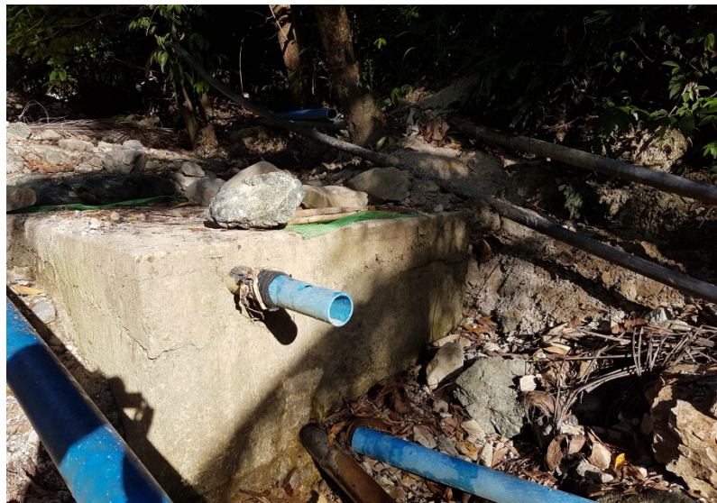
Figure 2. A closed type concrete intake box in Purok 7 in Barangay Balite constructed approximately 20 years ago. The Balite Creek supplies all seven (7) puroks except purok 1. The local residents now refuse to use this as their source of potable water.
