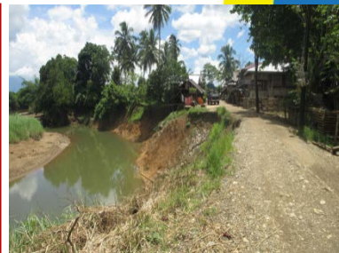
A riverbank erosion scouring a gravel-paved road in Purok Bacan-Bacan, Brgy. Layog affecting the gravel-paved barangay road and some houses nearby.
