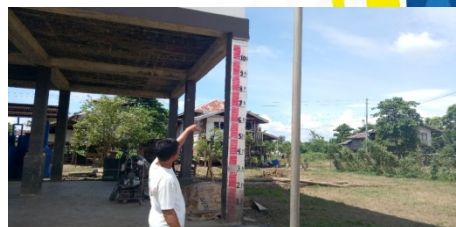
Photo showing the flood height markers on the post of Evacuation Center in Campo 6, Barangay Nueva Era were flood height reaches up to 9 ft.
