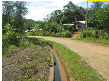
Drainage canals were installed along road sections of barangay Cuarinta, Dinagat
