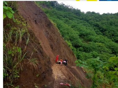
Road cut along Prk 5, Sitio Kahayagan, Brgy. Del Rosario, Sibagat, Agusan del Sur - named as "Taclaban" due to frequent landslide along the road due to very steep slope. rainfall.
