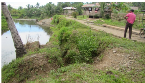
Active river scouring in Cagdao creek embankment spotted in Purok 5-B of Barangay Castillo. The observed scoured was almost hit the access road in the area. Geographic coordinates 8° 54' 53.6" North latitude 125° 57' 55.0" East longitude.
